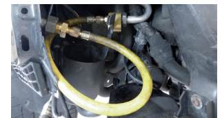
Figure 2: Filter-driers/accumulators should be bypassed and replaced before flushing.
